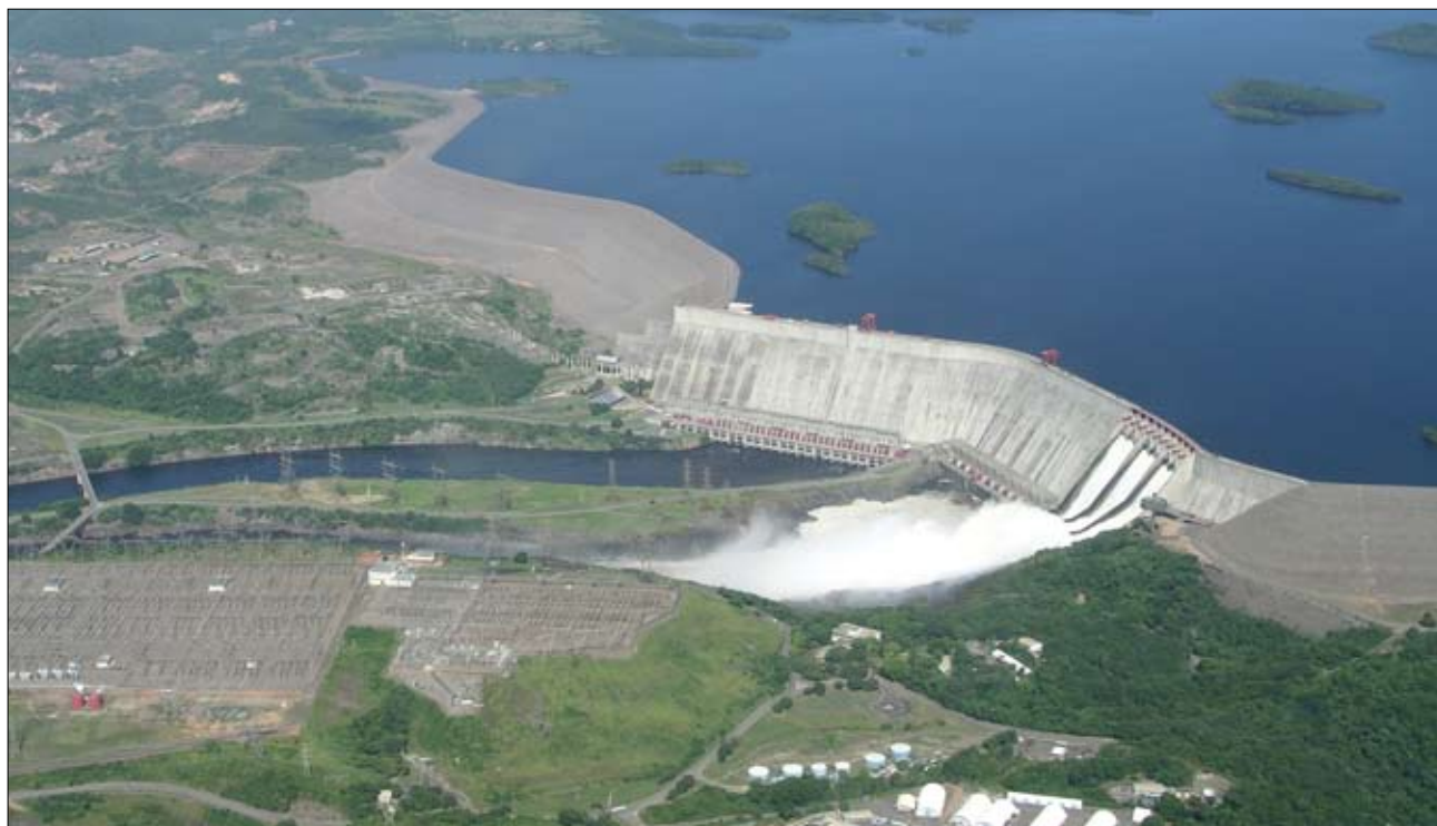
Figure 2.15. Large hydroelectric projects like the Raul Leoni Dam at Gurí on the Caroni River in Venezuela provide subsidized energy for aluminum smelters. Like many dams, it is situated near the mouth of a large river to maximize electrical energy production, which depends on water volume and vertical drop. However, placing the dam at the mouth of the river also isolates fish populations of the entire watershed from the rest of the Orinoco basin (© Daniela Vizcaino/CI).
